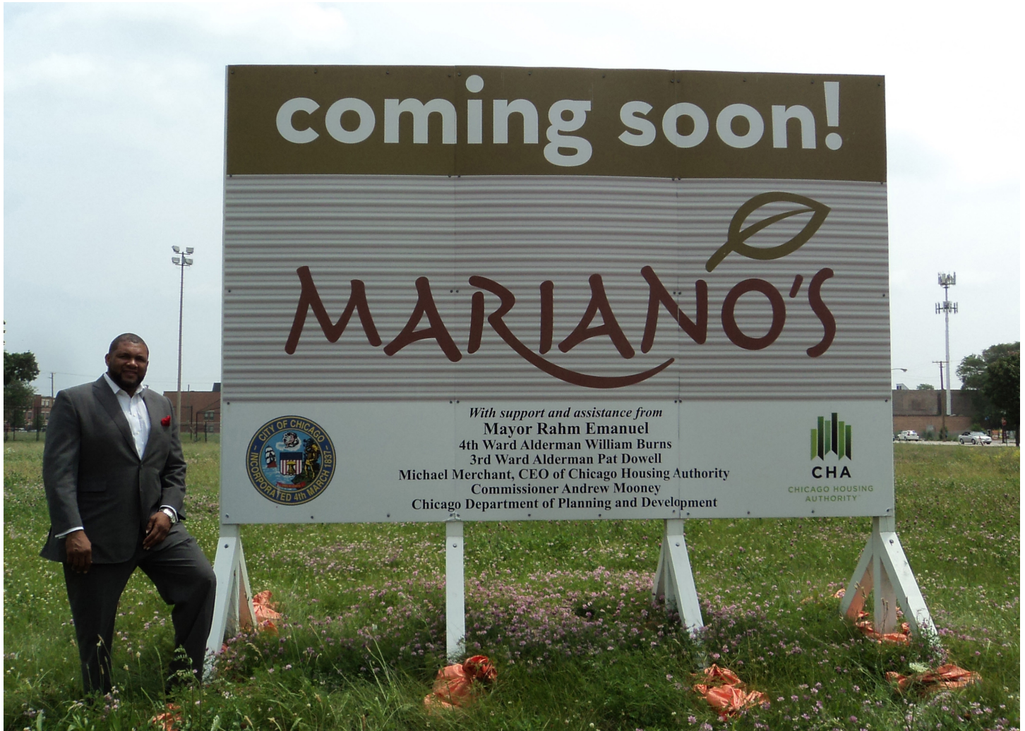
WILBUR C. MILHOUSE AT THE BRONZEVILLE MARIANO'S CONSTRUCTION SITE. MILHOUSE ENGINEERING AND CONSTRUCTION SERVED AS GENERAL CONTRACTOR ON THE PROJECT. THE 74,000 SQUARE-FOOT STORE OPENED IN OCTOBER 2016.
