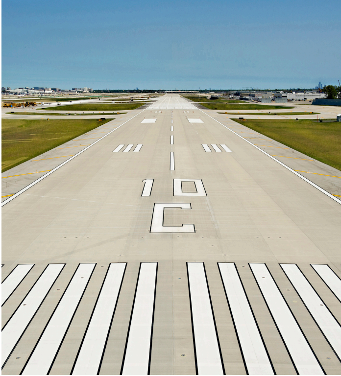
FINISHED RUNWAY 10C AT O'HARE INTERNATIONAL AIRPORT.
